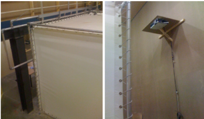
Figure 2; Physical installation of the CryVE system.
